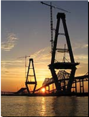
The bridge's 1,546-ft main span is supported by two 575-ft-high, diamond-shaped towers Source: constructorage.construction.com
