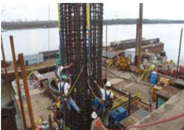
Insertion of rebar cage and O-cell assembly
